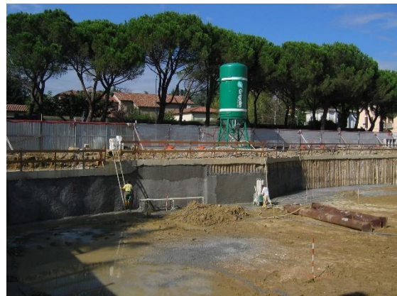
Spritz beton (mq 1.000) – Platee in c.a. (mc 1.300)
